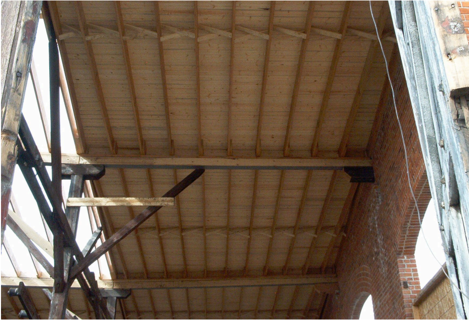
Decking over bay #8, looking toward the back of roundhouse.
